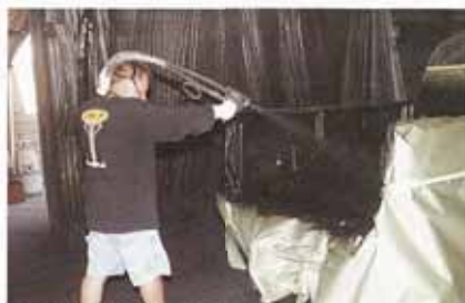
26. Mike hits the bed with several coats of Line-X, which will protect the bed when Bill hauls his tools to the job.
