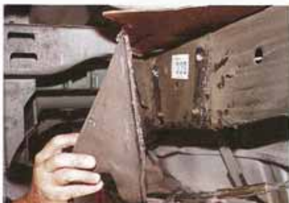
19. Using an air chisel remove the factory hanger from the frame.
