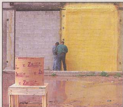
Workers made final preparations before detonating a 200-pound bomb (in foreground) to test blast mitigation coating developed by Line-X. The left side of the block wall was untreated.
