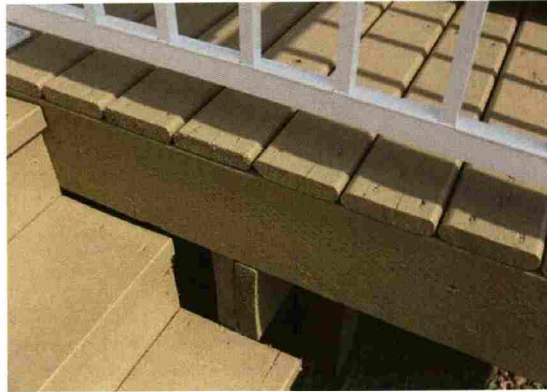
Outdoor decks and stairs get the treatment. Photo courtesy of Scorpion.
