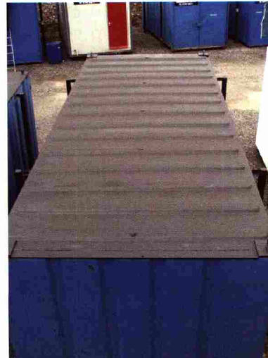
A portable cabin/storage unit can use a spray treatment to keep it waterproof. Photo courtesy of Qwik Liner.
